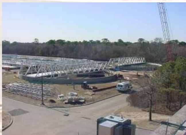
The primary clarifiers at the North Plant will be fully covered, enhancing OCUA's ability to control odors.
